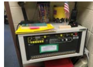
Intercom System Head-End
