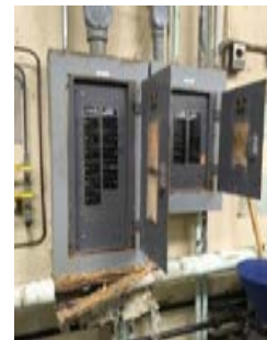
Corroded Panelboards
